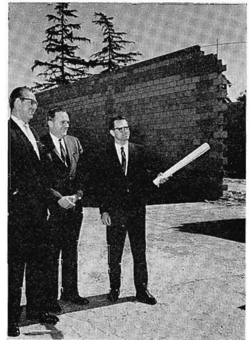
John K. West (left), RCA Staff VP, E. Robert Turner, Burbank City Manager, and Gordon W. Bricker, West Coast Operations Mgr., RCA, check building progress.
